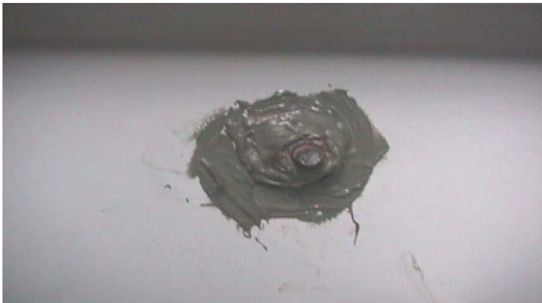
Non-factory putty keeps bolts in place.
