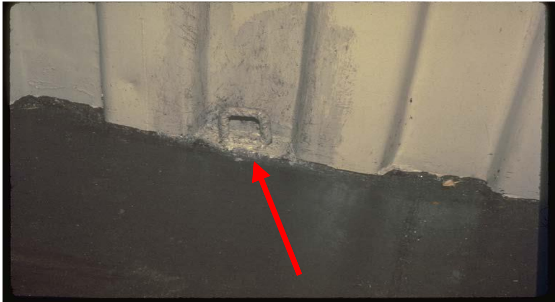
Sloppy repairs and welding.
