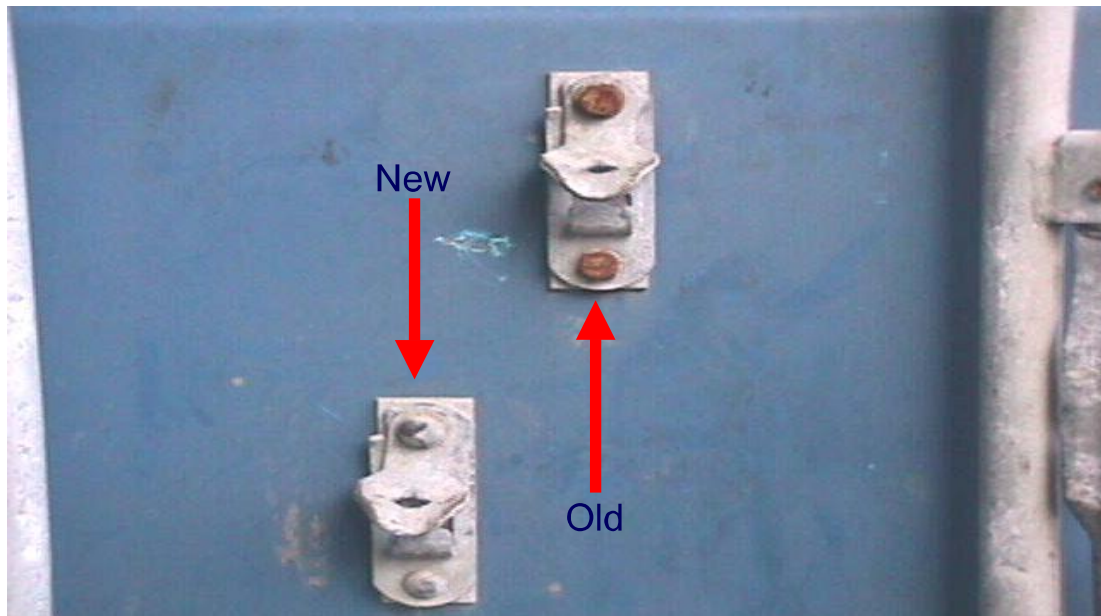
Rivet type & color/ New & old rivets together.
